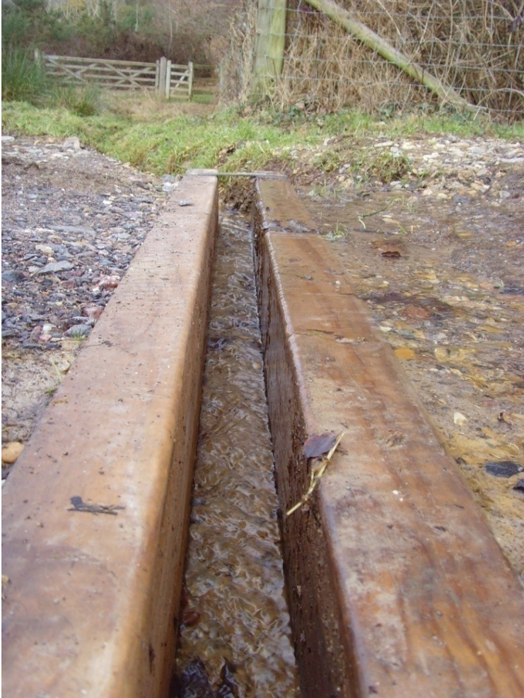
1 of 2 drainage ditches crossing the main track within zone 3
